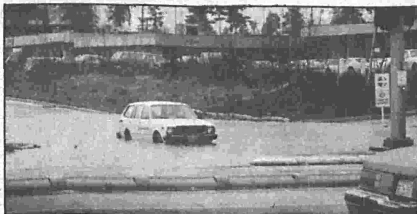
THE STRETCH of Pacific Highway South between South 320th and 326th streets seems to be more commonly recognized in this state than dry these days as torrents fill the street with rain runoff. The drainage system there is inadequate, county and state officials agree, but there is no immediate funding available for the project.
