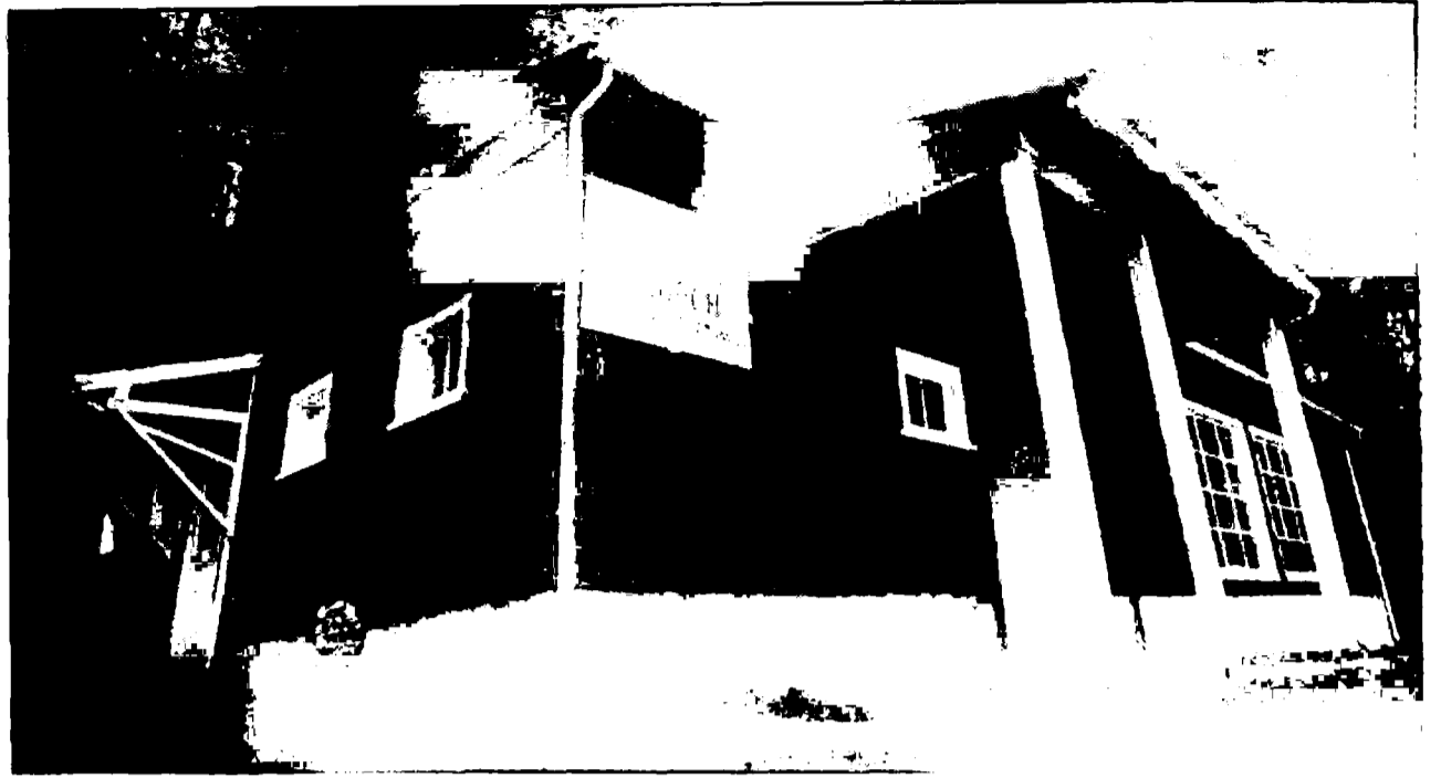
TODAY THIS BUILDING sits on the hill overlooking Puget Sound and serves as the only central meeting place in Redondo. It was built by the community's residents in the early 1940's, but what may become of the building within the next few years is a little uncertain. The Federal Way School District administration is considering selling the land because it no longer is useful to the schools.
