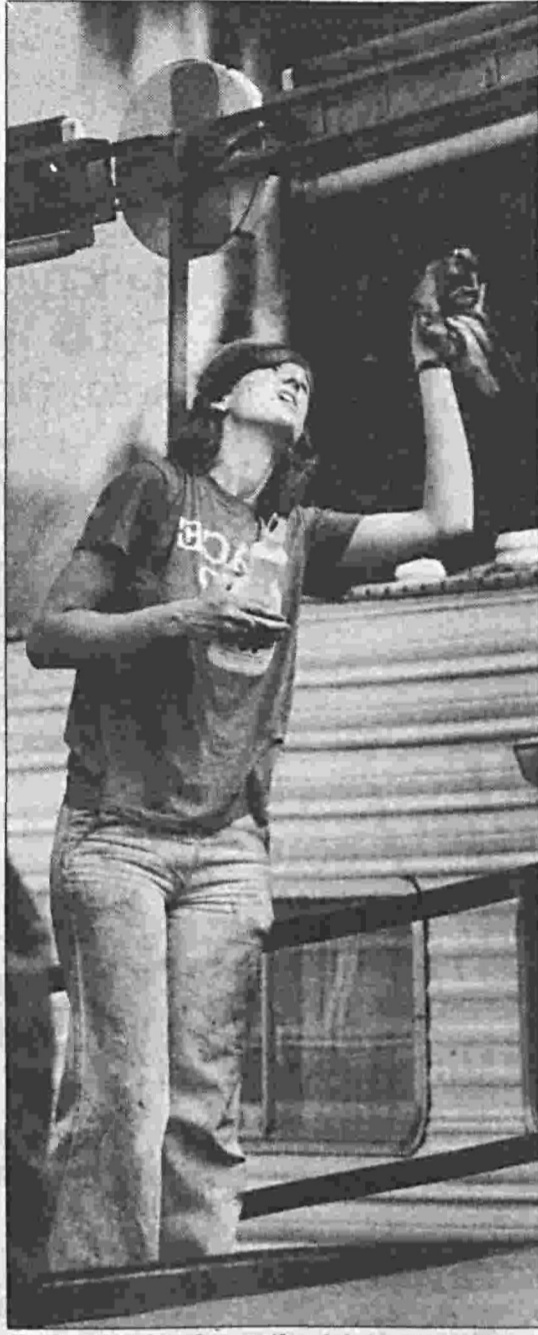
Kathy Splain cleans the joints of the ferris wheel with a degreasing solution.
